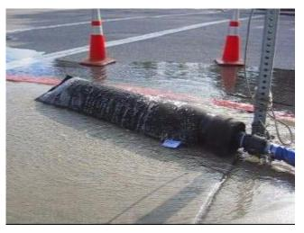
The EVAC Filtration System filters suspended solids as fine as rust and hydrocarbons
